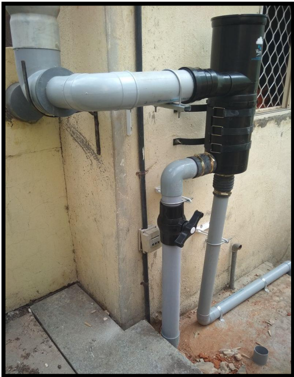
Rain Water used to recharge the Bore well
